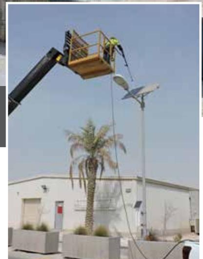
*We proposed installing solar street lights on Isa Air Base for energy savings. The 80 street lights provide an annual savings of over \$25,000, and an annual fuel reduction of 1,900 gallons. The simple installation of the lights was completed without disruption to the mission, the environment, or the infrastructure.*
